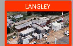
8-Ft High Temperature Tunnel** Large-scale Hypersonics & Propulsion
