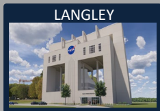
Flight Dynamics Research Facility Spin and Forced Oscillation -Under Construction-
