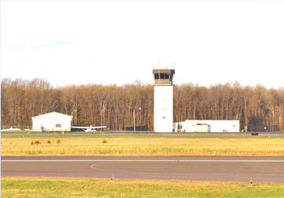
Existing ATC Tower
